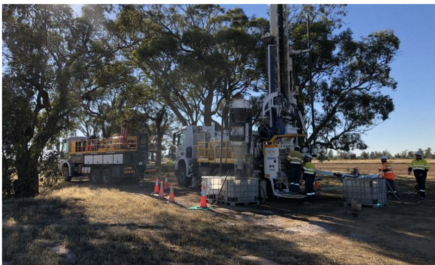
Drilling at the Pyramid Hill operation.
